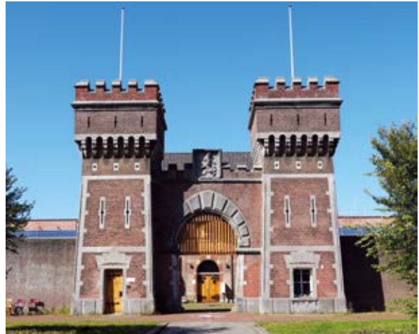
KSC Detention Facilities
